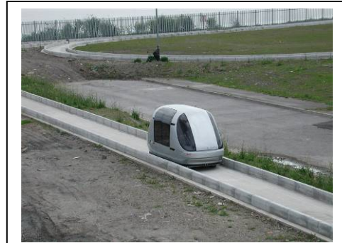
Figure 1. ULTra's at-grade open guideway.
